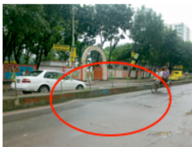
Fig.25 speed breaker in front of school present but hardly can be seen, due to the absence of proper road marking (showing two different well known schools at Mohammadpur)
