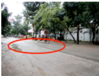
Fig.16 speed breakers can hardly be seen, which can cause accidents
