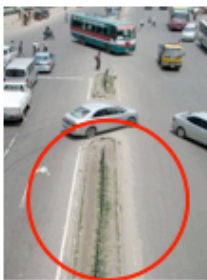
Fig.7 Road markings are very poor to read
