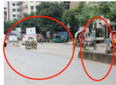
Fig.23 Absence of road marking along with no 'u-turn' signage
