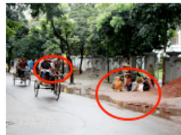
Fig.18 construction materials here and there without any safety measures
